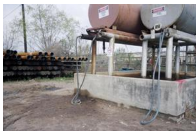
Insufficient bunding
