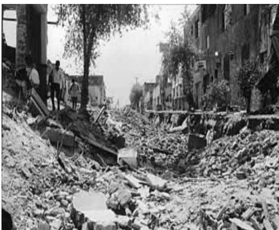
Rubble in center of street destroyed by sewer explosions in Guadalajara, 1992. Photo credit, with permission (Jon Seals): Disaster Recovery Journal at: http://www.drj.com/dnworld/content/w2_028.htm ; accessed May 5, 2006.
