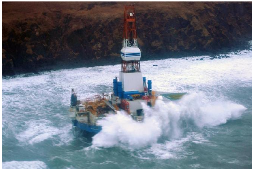
Picture: Waves crash over the conical drilling unit Kulluk where it sat aground on the southeast side of Sitkalidak Island, Alaska, Jan. 1, 2013. U.S. Coast Guard photo by Petty Officer 3rd Class Jonathan Klingenberg
