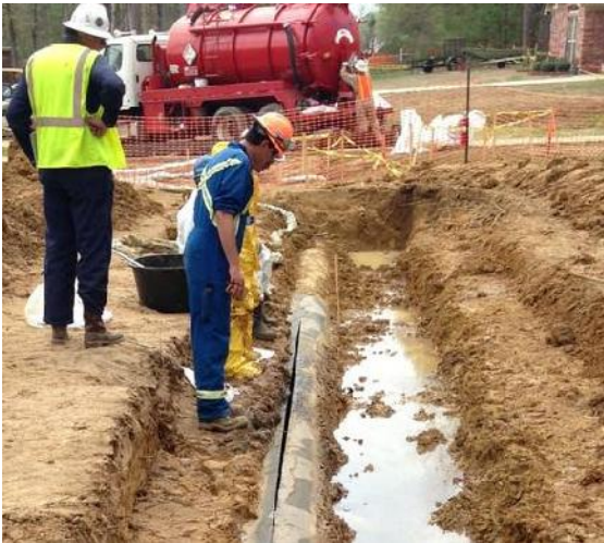
Photo: A 22-foot long rupture on Exxon Mobil's Pegasus pipeline sent around 200,000 gallons of crude oil into a residential neighborhood in Mayflower, Ark.
