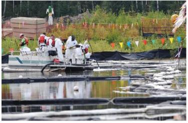
Canadian Natural Resources Limited (CNRL) workers cleaning up the bitumen emulsion on this marsh after it seeped up through a fissure under the water at their Primrose oilsand projects north of Cold Lake, August 8, 2013. A total of four sites have this seepage occurring and to date 7300 barrels have been collected from 13.5 hectares. Photograph by: Ed Kaiser, Ed Kaiser
