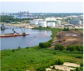
The Money Point site during dredging of PAH-contaminated sediments. The orange boom contains the released sediment. The VIMS scientists operated the biosensor from the small boat near the boom. Photo courtesy of Joe Rieger, Elizabeth River Project.
