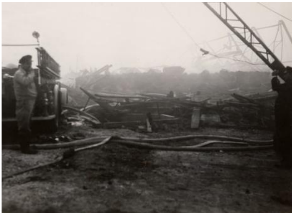
This barge, originally located near the explosion, was lifted out of the water and landed 100 feet inland. The firetruck at left (behind the man) was thrown there by the second explosion. Photo taken April 18, 1947. (Courtesy of Special Collections, University of Houston Libraries. UH Digital Library)
