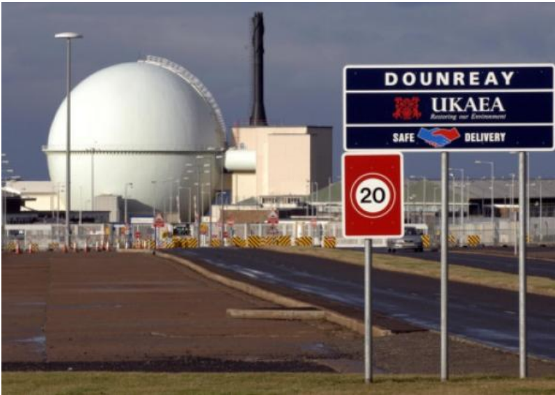
Dounreay nuclear power station in Caithness. Picture: Ian Rutherford
