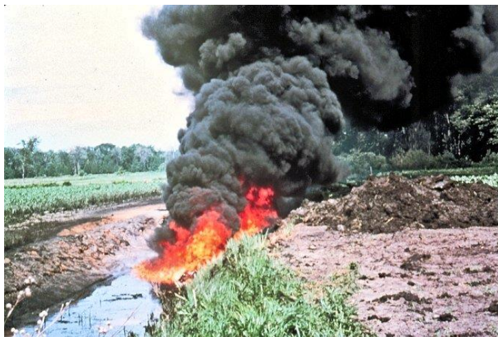
Figure 34 Burning of a fuel oil spill in a drainage ditch. This is a frequently-used technique to deal with such spillage.
