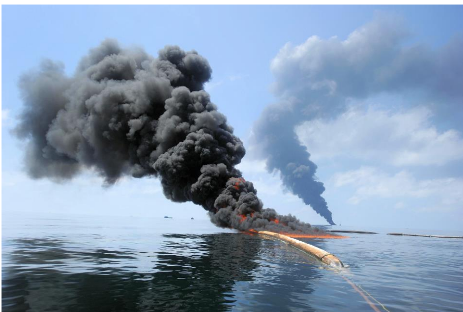
Figure 38 Heavily weathered oil is burned inside a fire-resistant boom during the Deepwater Horizon Spill. Another burn is far in the background.
