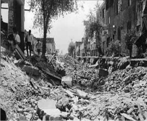
Rubble in center of street destroyed by sewer explosions in Guadalajara, 1992. Photo credit, with permission (Jon Seals); Disaster Recovery Journal at: http://www.drj.com/drworld/content/w2_028.htm ; accessed May 5, 2006.
