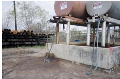
Insufficient bunding
