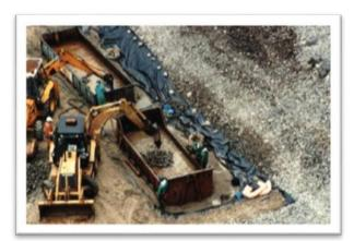
Oil could then be skimmed off the surface of the pit and the cleaned cobbles returned to the beach.
