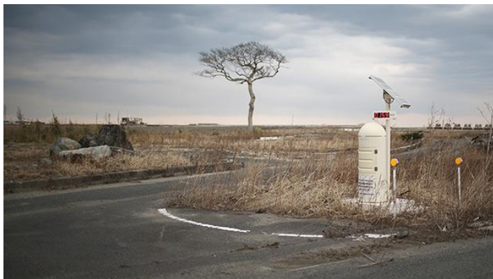
Photo: Christopher Furlong/Getty Images A radiation monitoring station alongside a road in Namie, Japan.
