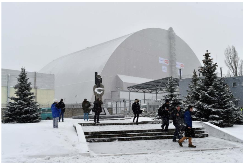
Picture: An arched shelter was slid into place over the Chernobyl nuclear disaster site in Ukraine on Tuesday. It is about 500 feet long, has a span of 800 feet and is 350 feet high. Credit Sergei Supinsky/Agence France-Presse — Getty Images
