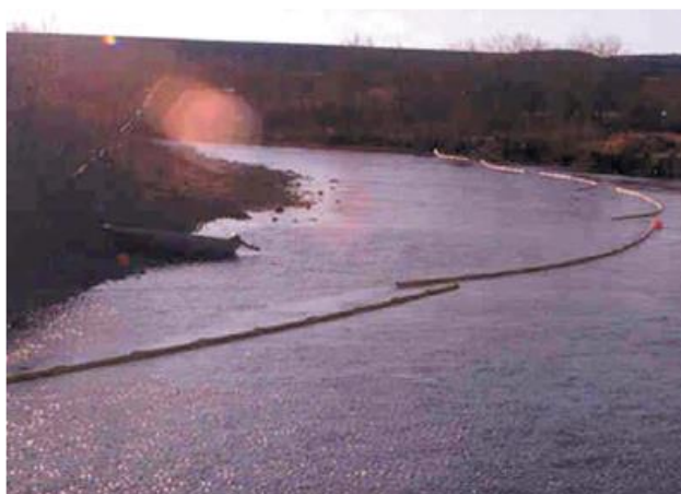
Photos: Below left, booms used to divert oil to a collection point; Below right, a deflector is used to position the boom at the desired angle
