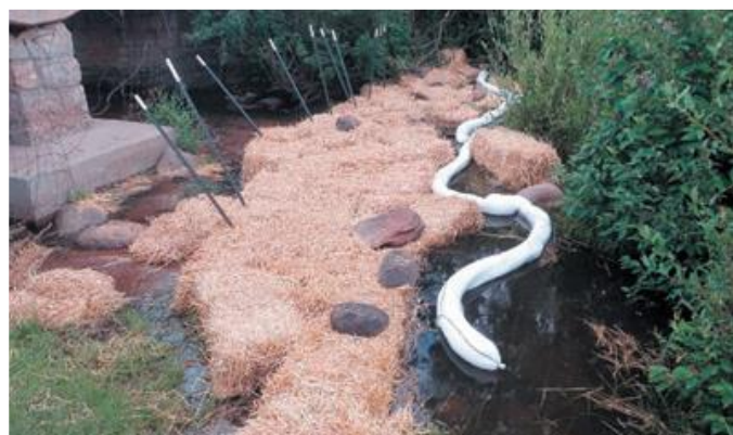
Below left: straw used to hold back and absorb low quantities of oil. Below right: oiled straw is disposed of by burning on site.
