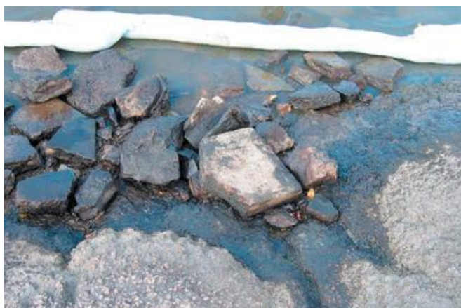
Below Left: Flushing oiled riprap after soak time.
