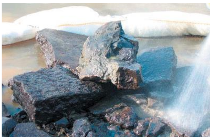
Below Left: Flushing oiled riprap after soak time.
