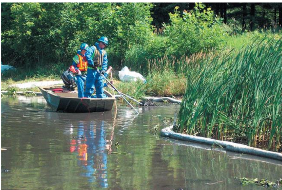
Above: Pumping water into river sediment to release sunken oil and flush it to the surface.
