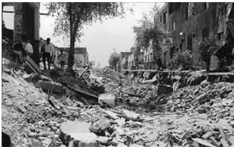
Rubble in center of street destroyed by sewer explosions in Guadalajara, 1992. Photo credit, with permission (Jon Seals): Disaster Recovery Journal at: http://www.drj.com/drworld/content/w2_028.htm ; accessed May 5, 2006.
