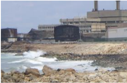
Jiyeh Power Plant (2006) ©REMPEC (2012)
