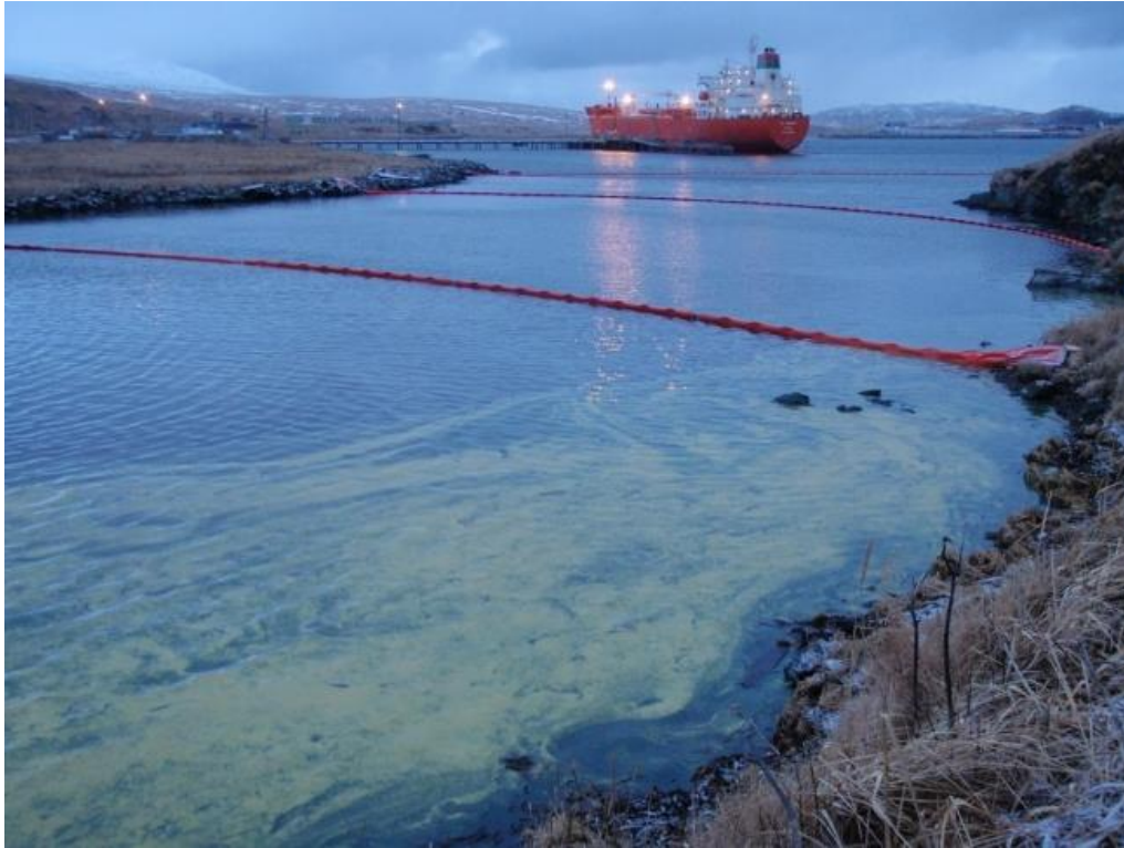
Diesel accumulating behind the first row of pollution boom after an oil spill in Alaska's Aleutian Islands in 2010. Image credit: U.S. Fish and Wildlife Service.
