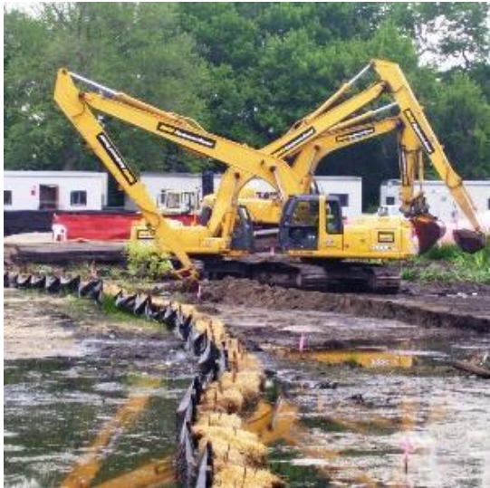
Liberty industrial finishing sediment dredging. Image credit: U.S. Geodetic Survey.
