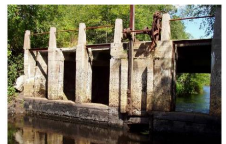
Horseshoe Dam before it was removed.
