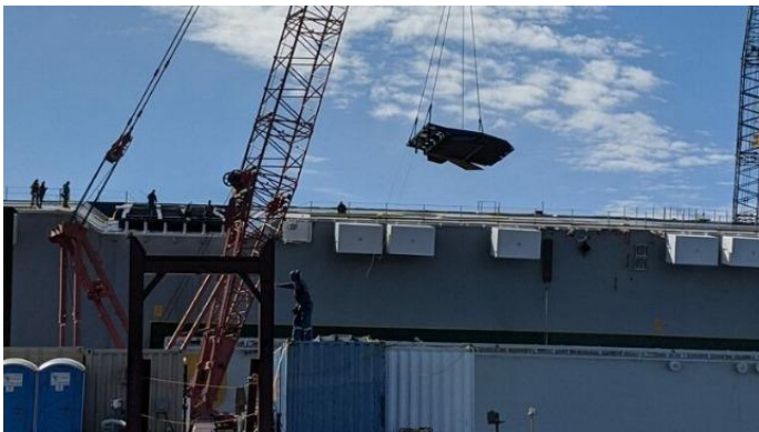
Photo: Ramp being removed from Golden Ray, credit: Coast Guard Petty Officer 3rd Class James Himes
