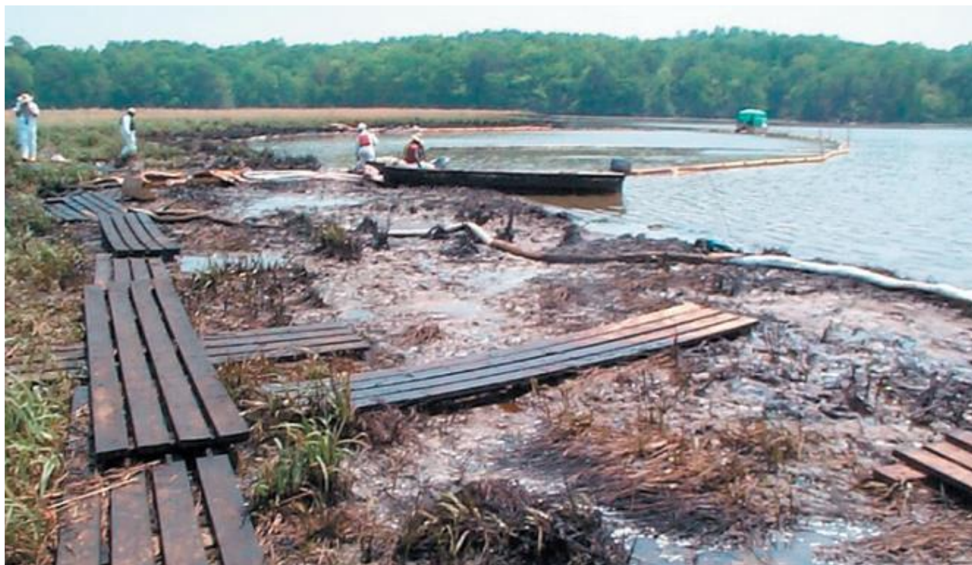
Above: Removing oil from a wetland contaminated with heavy fuel oil — planking is used to reduce trampling.
