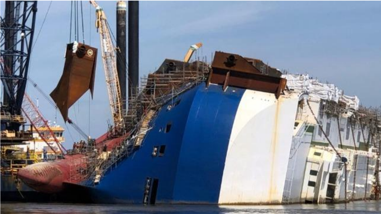
Above: Installing a lifting lug on Golden Ray's hull, June 2020 (St. Simons Sound Unified Command)
