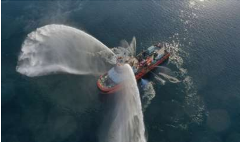
Photo: KOC Al Zour tests its fire-fighting system (source: RAL)
