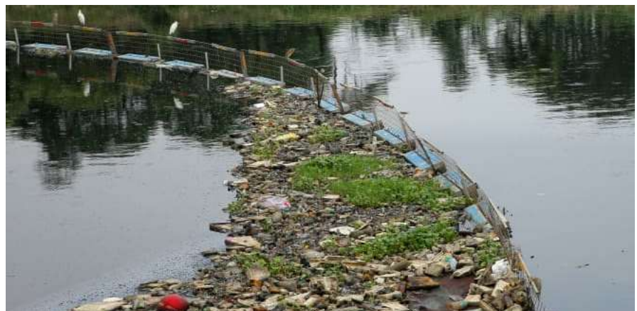
The AlphaMERS floating barrier captures trash as it flows downriver Photo from AlphaMERS
