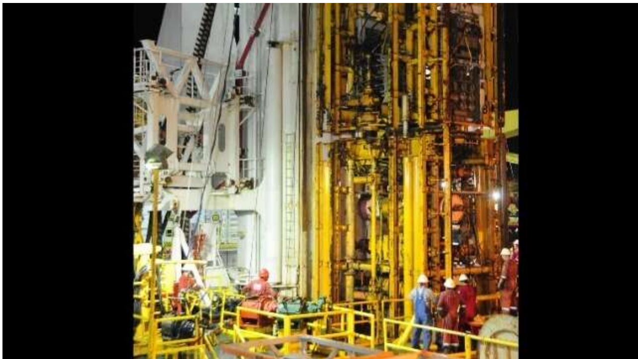
The regulations were born out of the failure of the Deepwater Horizon's BOP stack (center right) in 2010 (USCG image)
