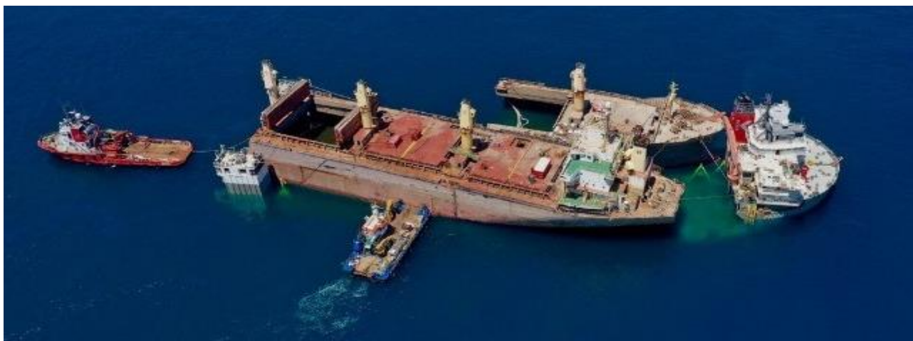
OS 35 bulker clearance Two sections of the bulker are now out of the water aboard a heavy lift vessel (Gibraltar Port Authority)
