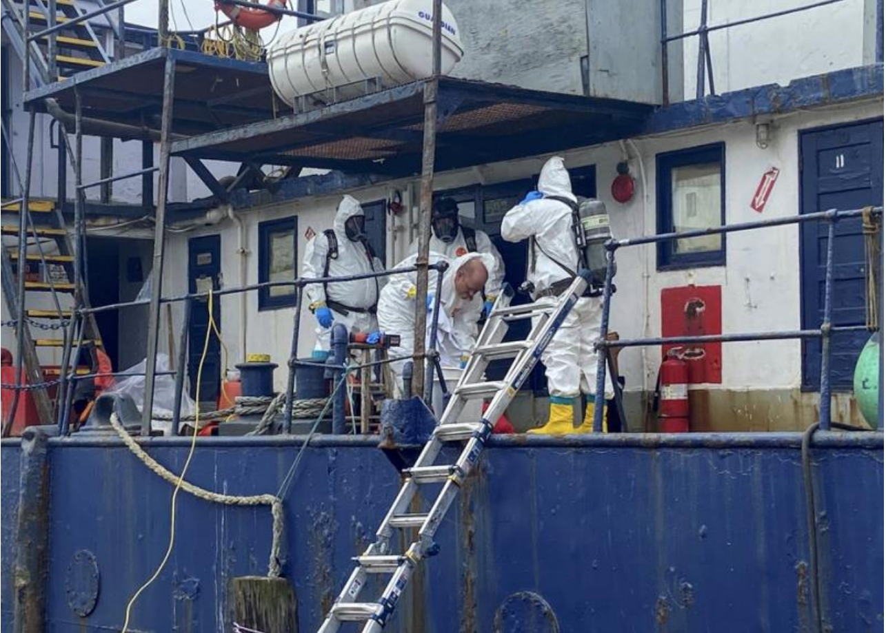
Above: Contractors in hazmat suits prepare to enter the fishing vessel Pacific Producer in Tacoma, Washington, on Sept. 1, 2023. Coast Guard crews from Sector Puget Sound worked with contractors to ensure all fuel, oil, and hazmat materials were removed. Image credit: USCG.
