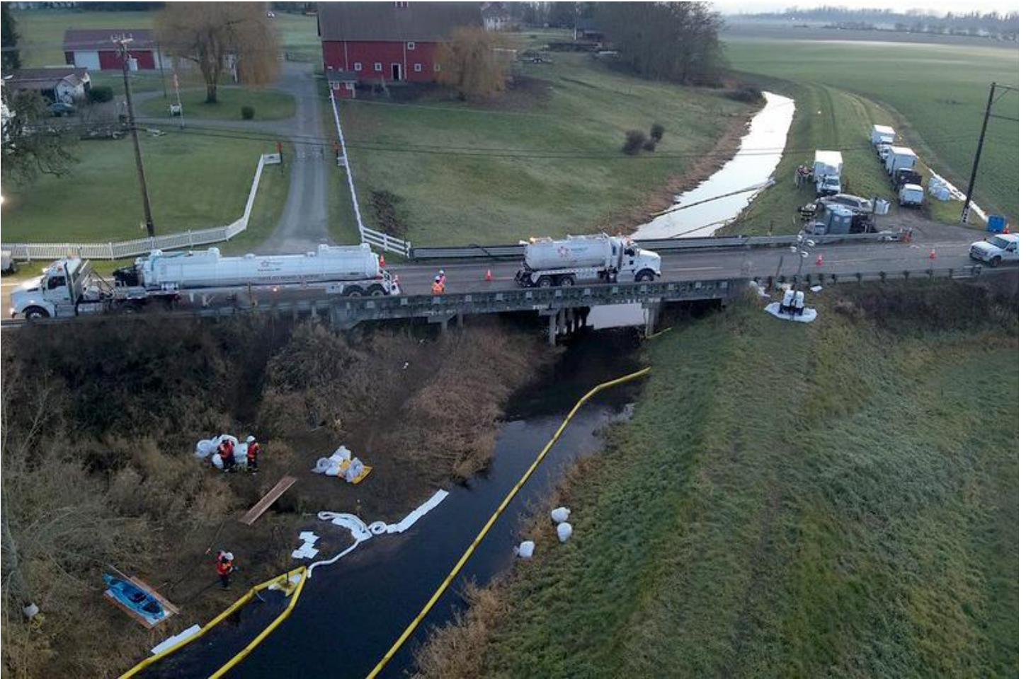
Above - The Olympic Pipeline spill emergency response in Conway, WA. Photo shows Hill Ditch and SR 534 looking south. The boom in the lower left of the photo is capturing the spilled gasoline for collection by a skimmer connected to the vacuum trucks parked on the bridge. Image credit: Washington Department of Ecology.
