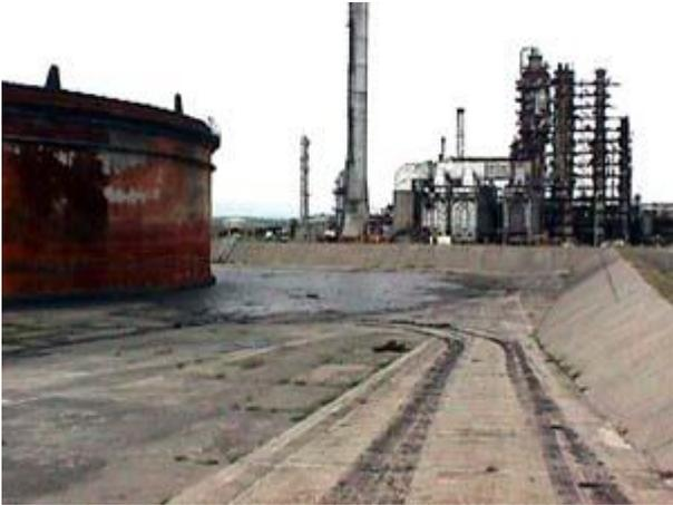
Surface containment: Purpose: to prevent the spread of oil on the surface and to prepare it for recovery.
