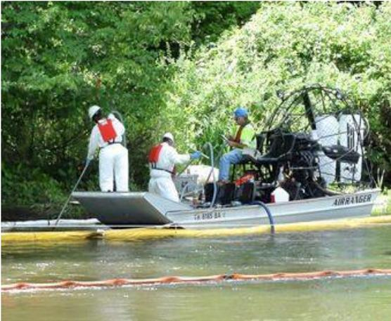
Workers pump jets of water into the riverbed to remove submerged oil from the Kalamazoo River, June 2011. Credit: U.S. EPA
