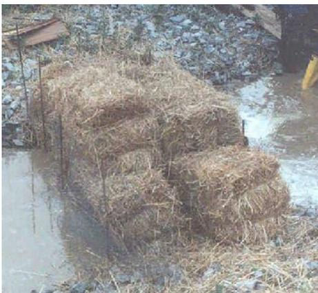
It needs to be said that the straw bale dam is very temporary as the straw absorbs large quantities of water and the bales *left* are tied with two thin polypropylene strings and are designed to be handled dry.
