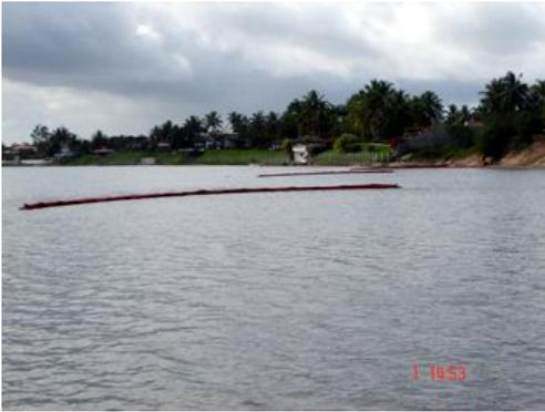
In order to reduce the stress and strain on boom anchor points a series of booms are positioned one behind the other to work like a cascade allowing the oil to be directed into calm water recovery points *photo left*.
