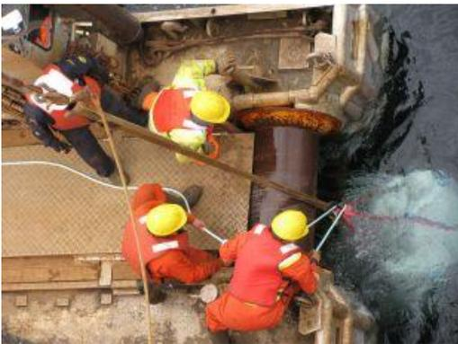
*Photo: A weighted neoprene gasket is manoeuvred from the Canadian Coast Guard Ship Anne Harvey to a smaller work barge for subsea placement to prevent oil from leaking from the Manolis.*
