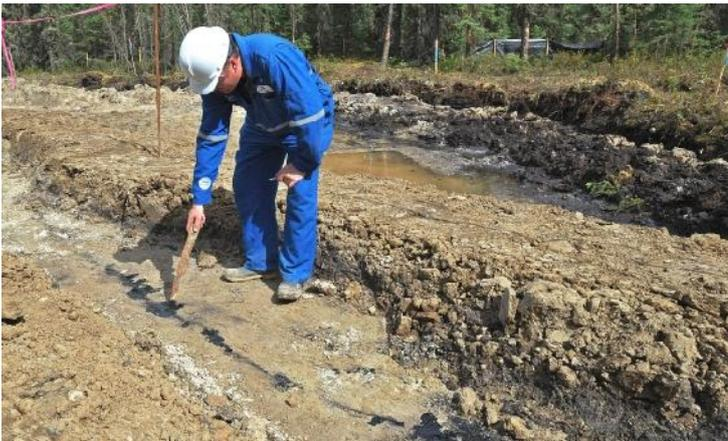
*Photo: Ryan Cameron, in charge of the cleanup, points to the bitumen emulsion seeping up through this fissure at Canadian Natural Resources Limited (CNRL) Primrose oilsand project sites north of Cold Lake, August 8, 2013. A total of four sites have this seepage occurring and to date 7300 barrels have been collected from 13.5 hectares. Photograph by: Ed Kaiser, Edmonton Journal*
