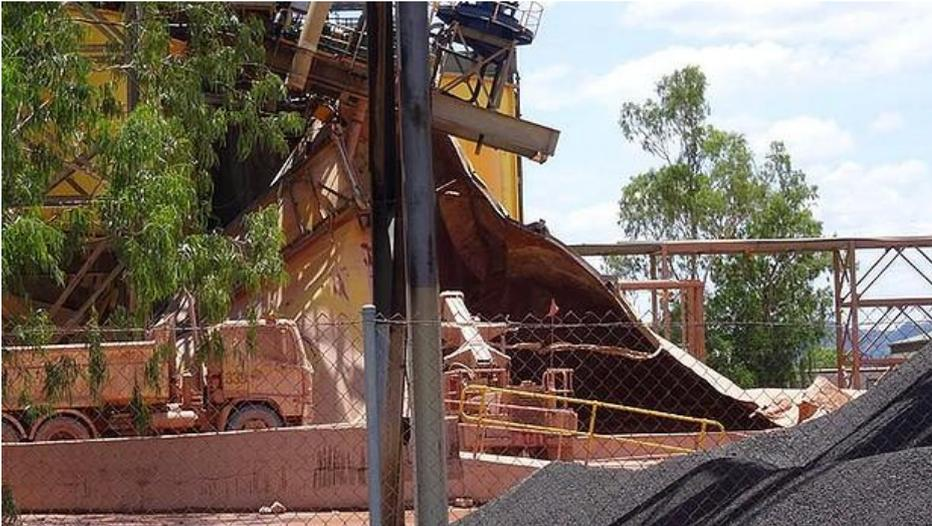
*Disaster: A truck and crane are swamped by acid slurry. All personnel were evacuated before the tank burst. Photo: Gundjeihmi Aboriginal Corporation*
