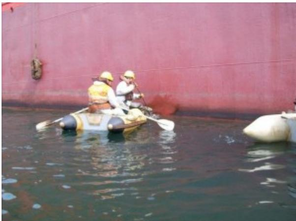
*12 vessels and the whole dry-dock were cleaned using Desolvit in conjunction with steam, absorbents and skimmers, allowing approximately 10 tons of oil to be collected from the surface*
