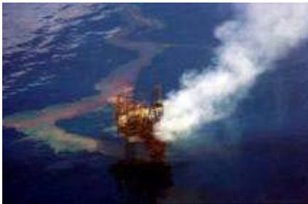
*Timor slick: oil and condensate leaches from the Montara wellhead platform days after the blowout*
